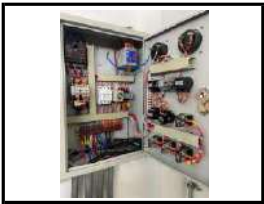
Pump Control Panel
