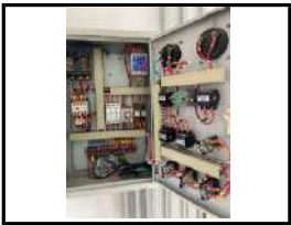
Pump Control Panel
