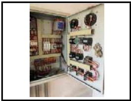
Pump Control Panel
